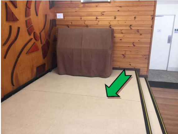
Photo 7. Interior, hall stage, cream floor coverings – non asbestos-containing sheet vinyl.
