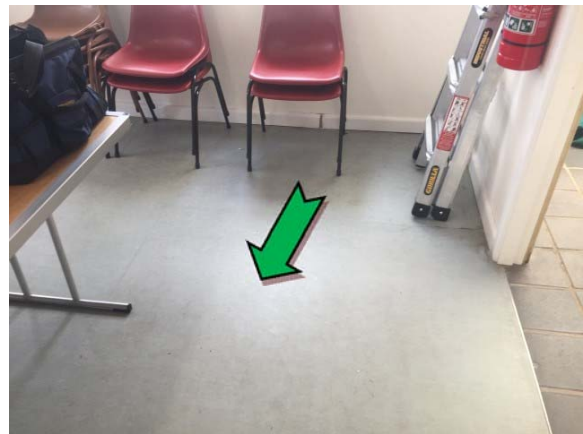
Photo 4. Interior, meeting room, light blue floor coverings – non asbestos-containing sheet vinyl.
