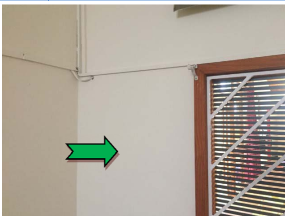
Photo 5. Interior, quiet room, southern wall – non asbestos-containing fibre cement sheeting.
