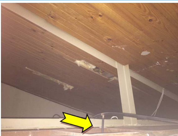
Photo 11. Interior, roof space, throughout, insulation – suspected SMF insulation batts.
