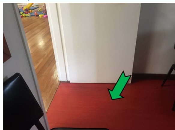
Photo 6. Interior, quiet room, throughout, red floor coverings – non asbestos-containing sheet vinyl.
