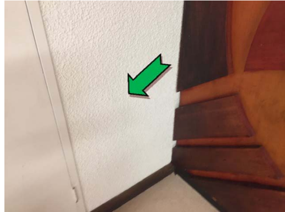
Photo 8. Interior, hall, eastern and northern elevation, walls – non asbestos-containing textured coatings.
