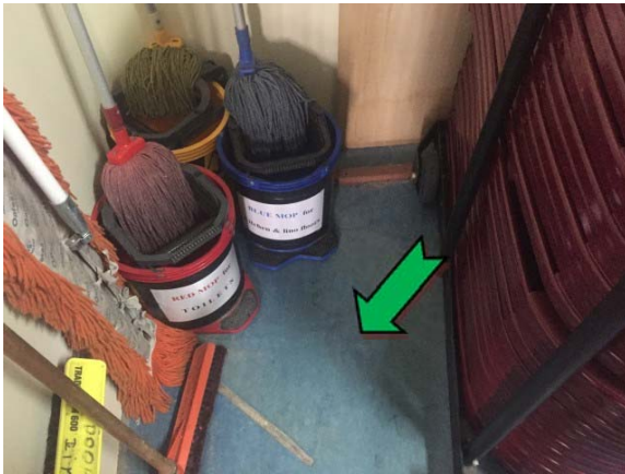
Photo 9. Interior, western store room, blue floor coverings – non asbestos-containing sheet vinyl.
